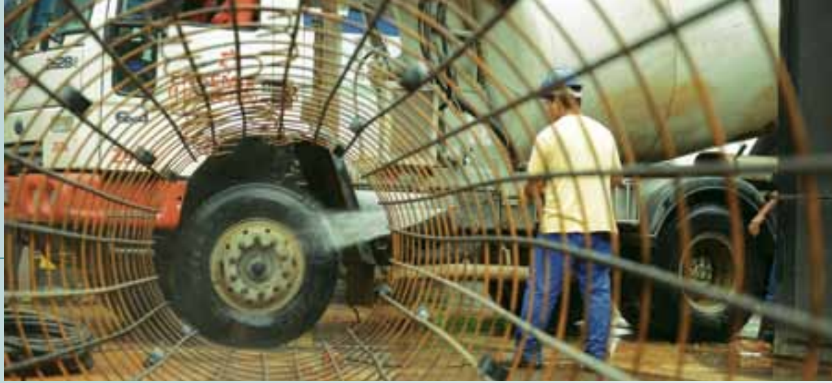
Cleaning Concern surrounding the works - “Lava Rodas” project
